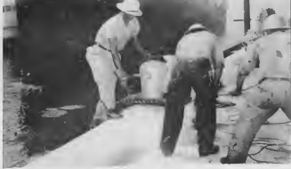
The Esso Marcester was the first ship to use the new Fl. 6,000,000 finger pier December 10. Nicolas Cues (left), assisted by two wharfingers, is shown slipping the first line over a ship's own mooring bit on the deck. (See next issue for a full account of the new pier.)
